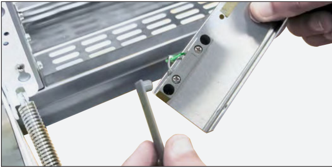
FIG. 4. Remove the plastic cover.
