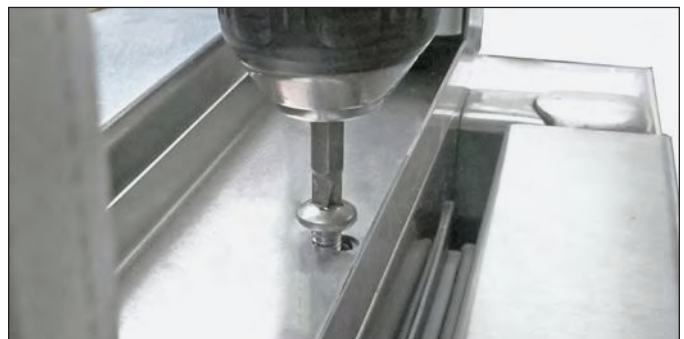
FIG. 10. Remove the screws from the metal channel.
