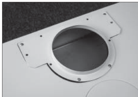
1. Remove pre-mounted 6" transition adapter or duct opening.
