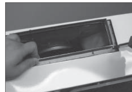
6. Mount starting collar (provided) at rear discharge.
