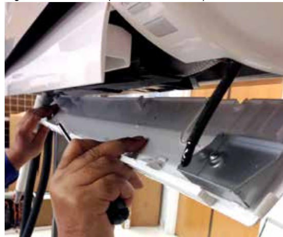
Figure 59: Remove (and Reattachment) Bottom Panel
