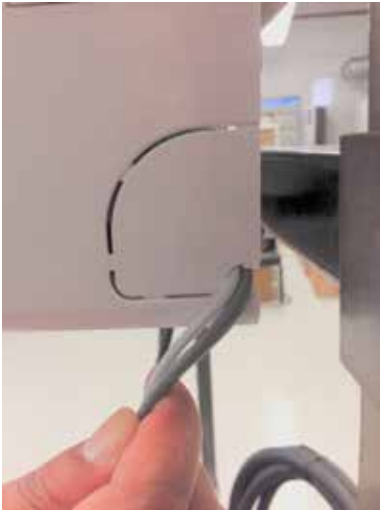
Figure 60: Indoor Unit Knockout (Communication Wires)
