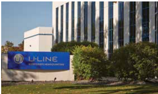
U-Line, Milwaukee, Wisconsin, USA
