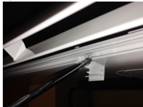
Figure 82: Remove (and Reattachment) Bottom Panel
