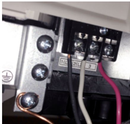
Figure 84: Indoor Unit Terminal Block with Grounding Cable (Example Only)
