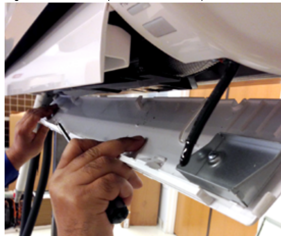
Figure 82: Remove (and Reattachment) Bottom Panel
