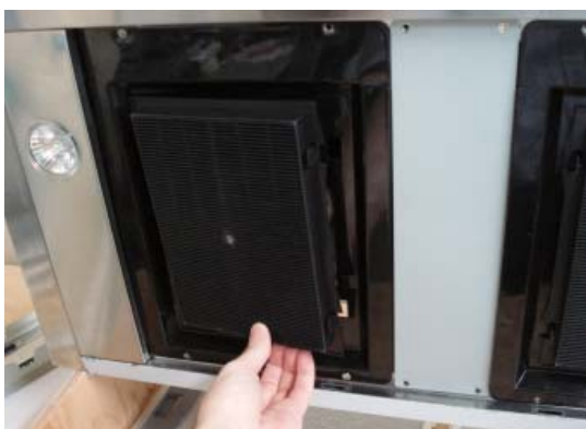
4. Install charcoal filters into charcoal filter brackets
