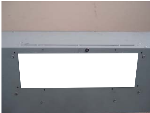
Horizontal Ducting (3-1/4"x10" Rectangular)
