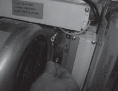
5. Remove existing grounding screw and attach grounding wire from capacitor box.
