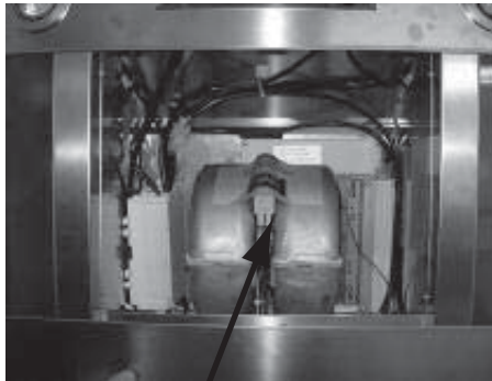
10. Remove wood block Final view of internal blower install.
