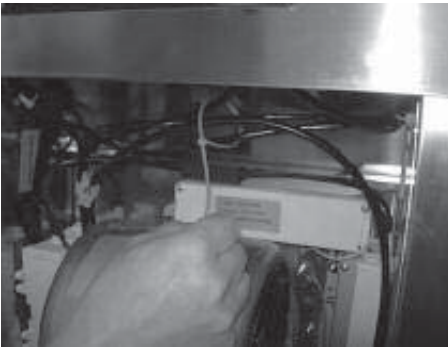
9. Use plastic tie to hold wiring together.
