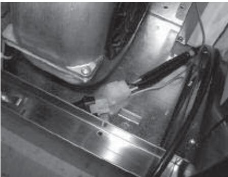
7. Attach short capacitor connector to blower connector.
