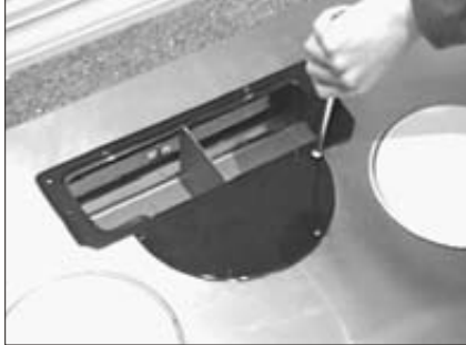
Option 2: (for flush cabinet base) Mount rectangular transition piece at opening with gasket as shown.
